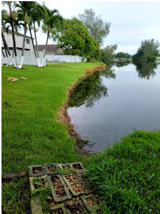
Embankment Restoration - Before
