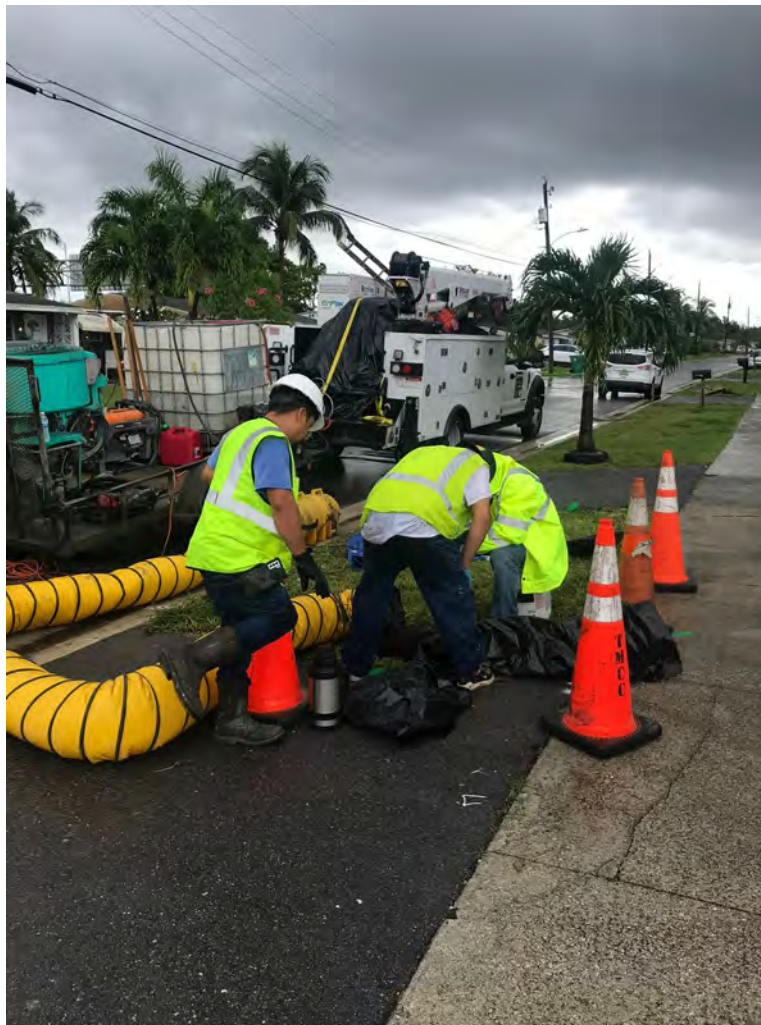
Critical Rehabilitation Work on a Manhole
