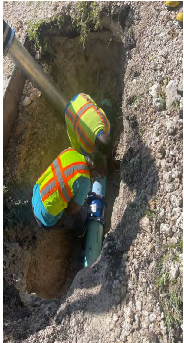
Main Break Repair by Staff
