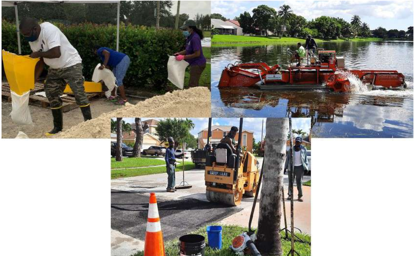
Public Works Crews - Sandbag Filling/Canal Cleaning/Roadway Repairs
