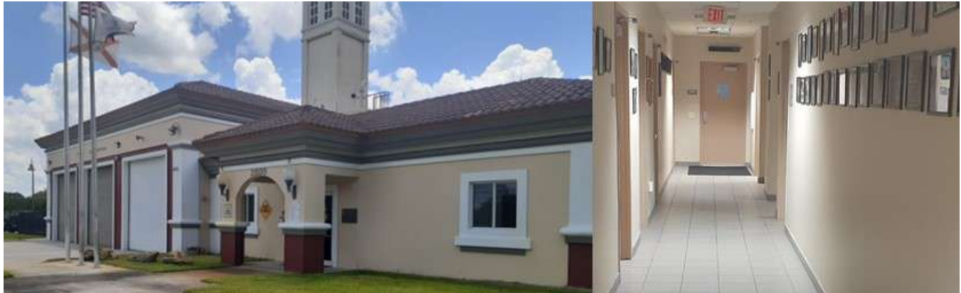
Building Maintenance - Interior & Exterior Repainting of Fire Station 100
