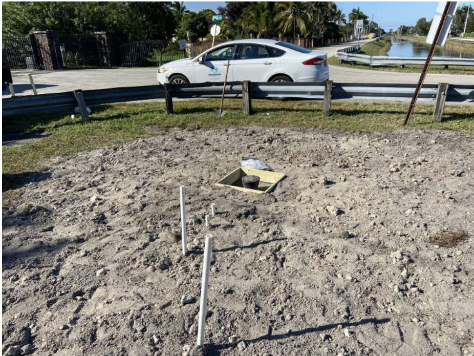
Completed utility work at Country Club Ranches
