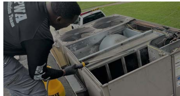
Staff Cleaning HVAC System at Fairway Park
