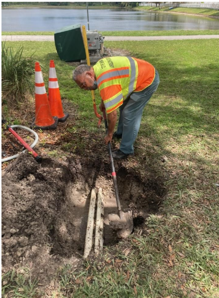
Excavating Irrigation Pipes
