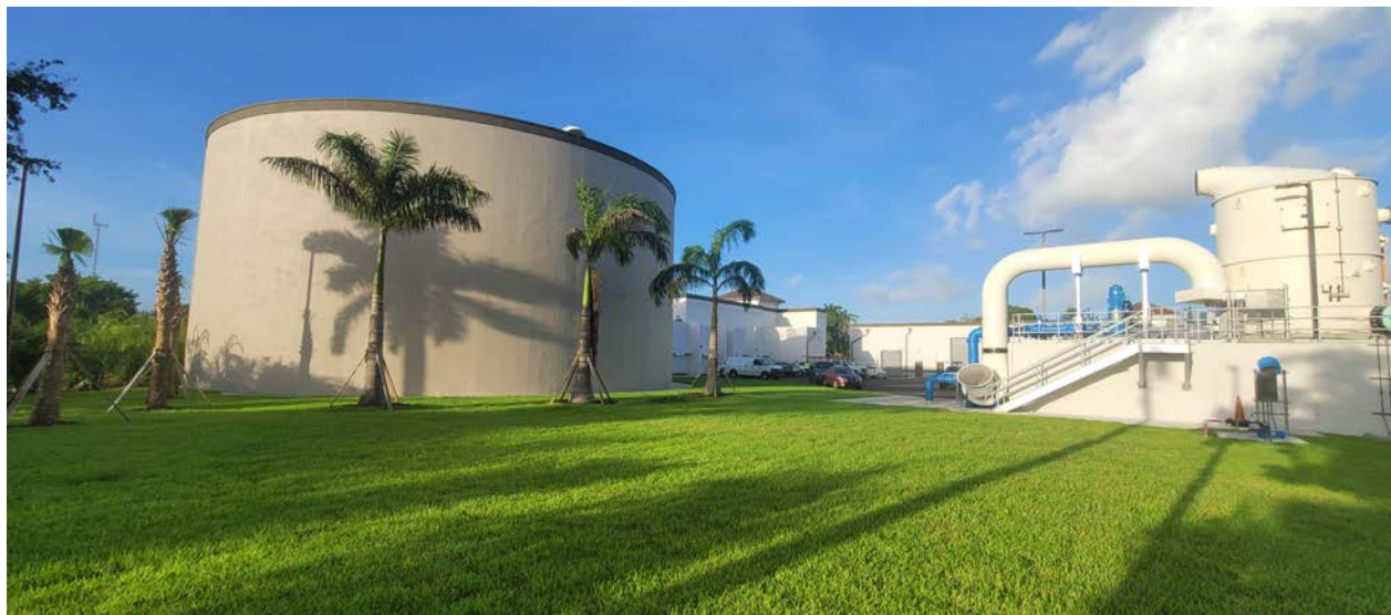
East Water Treatment Plant New Ground Storage Tank for Treated Water
