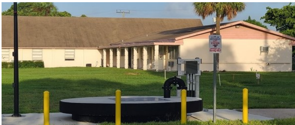
A Completed CIP Project - Historic Miramar Infrastructure Improvements
