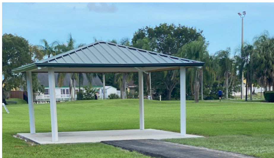
The construction of a new pavillion was completed at River Run Park as part of the Capital Improvement Program.
