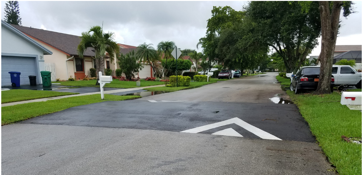
Speed Humps are installed to control traffic speed; therefore keeping neighborhoods safe.
