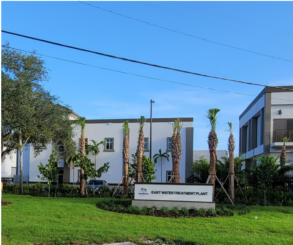
The East Water Treatment Plant of the City of Miramar.
