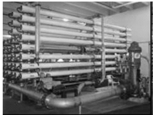
(b) Nanofiltration at West WTP
