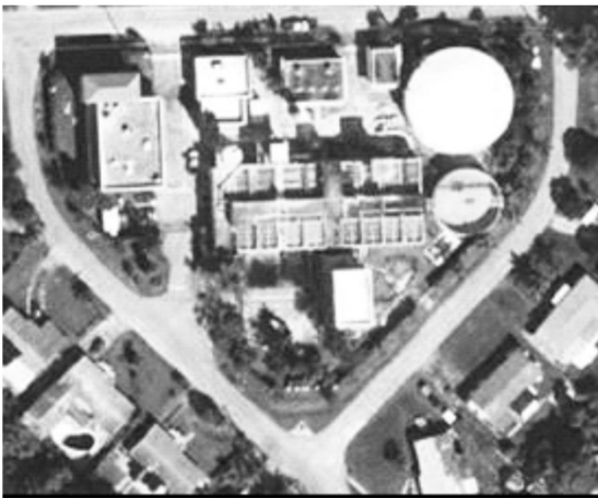
(a) Aerial View of East WTP
