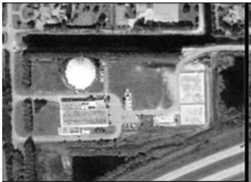
(a) Aerial view of West WTP
